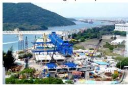
The HKLR comprises a 9.4km long viaduct section going from the HKSAR boundary to Scenic Hill on the Airport Island. The design was using segmental box girders and erected in balanced cantilever method. The decks were formed by 3 single box girders or 2 single box girders with stitching together. The single bored pile was used as foundation without pile cap.
